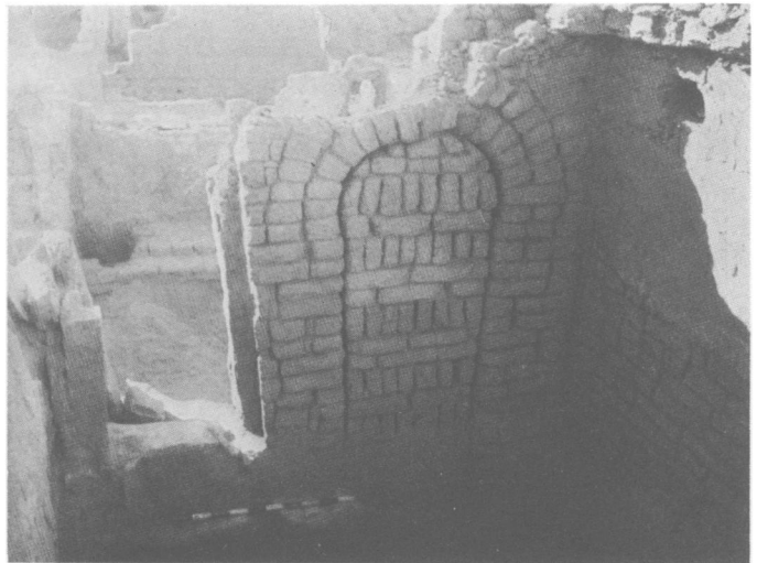
4. Blocked doorway in building E.13.2. AAe
